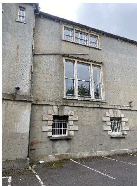
Fig.20: North elevation, core house. Square-headed window openings with 2 no. mullions and Square-headed windows with bossage surround to basement.
