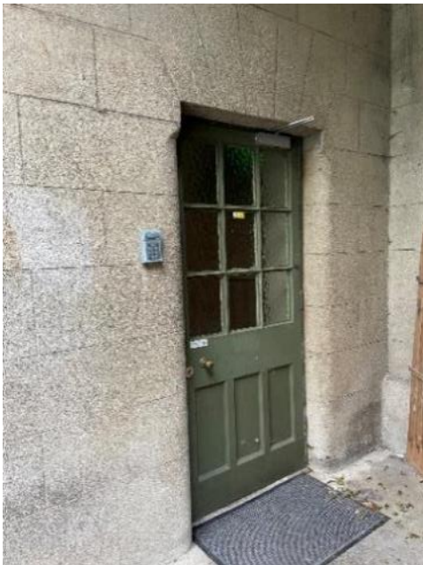
Fig.23: North elevation. Square-headed door opening.
