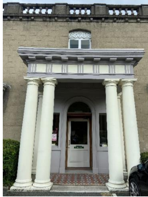
Fig.22: South elevation. Doric entrance portico with ceramic tiles finish. Round-headed door opening.
