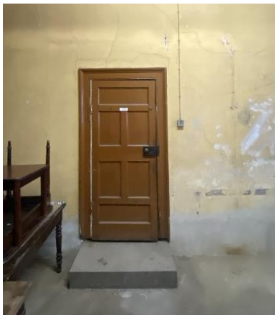
Fig.106: B-22, historic door architrave
