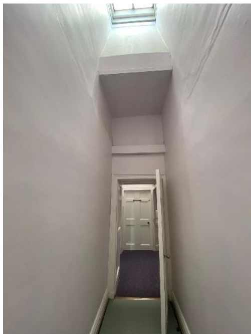
Fig.85: View facing south, rooflight
