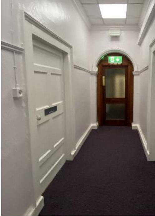
Fig.110: 1-37, historic six panel timber door
