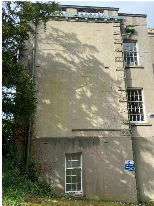
Fig.18: East elevation, 20th C wing with ruled and lined cementitious render.
