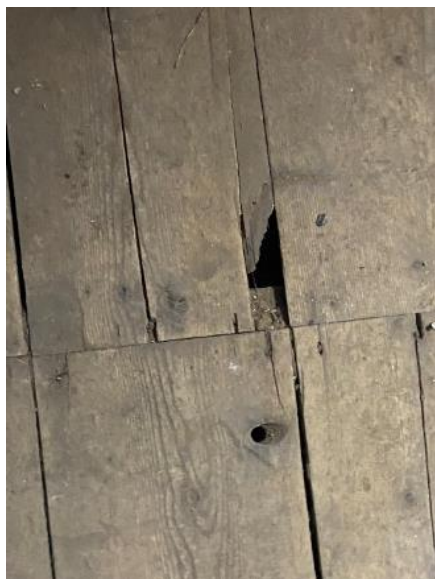
Fig.104: B-21, historic timber floorboards, missing section and gaps between the boards.
