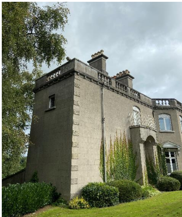
Fig.17: West and north elevations, 19th C wing with ruled and lined cementitious render.
