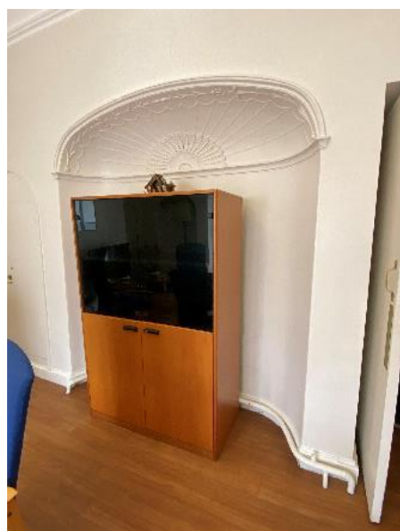
Fig.60: North wall, alcove with plasterwork
