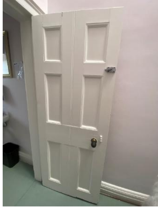
Fig.111: 1-22, historic four panel timber door
