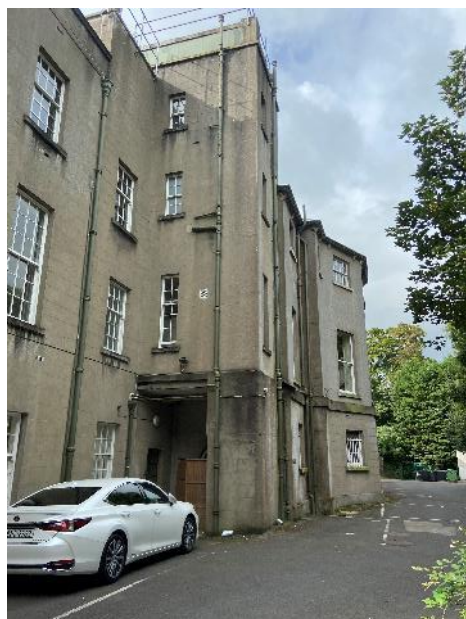
Fig.17: West and north elevations, 19th C wing with ruled and lined cementitious render.
